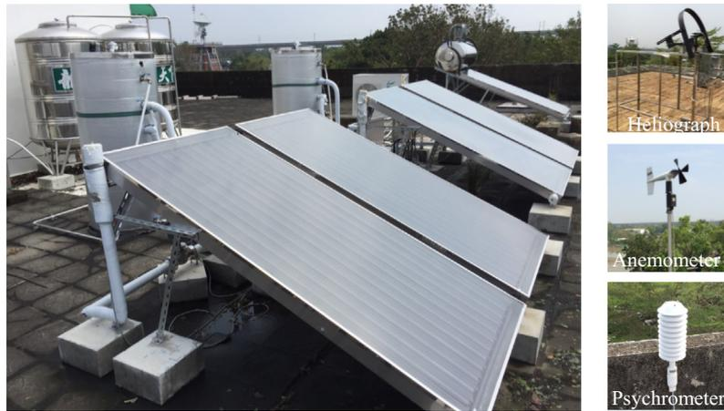
Fig. 1. Photograph of the solar domestic hot water demonstration system with environment detection sensors.
